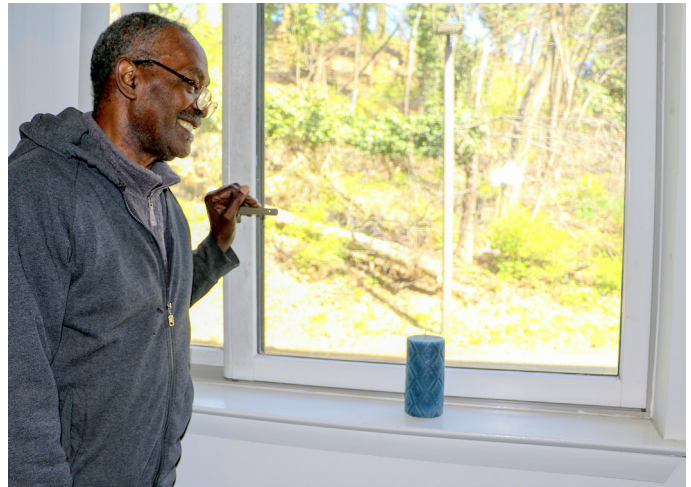
Resident Alvin Williams gazes out one of the 28-year-old windows at St. Joseph's Villa. "You can really feel a draft on cold days," he says. The replacement of these windows is essential to Resident comfort and safety.
